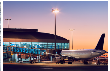
High Mast Lighting
